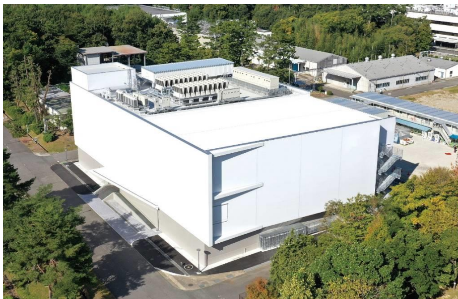
External views of the 5th manufacturing building
