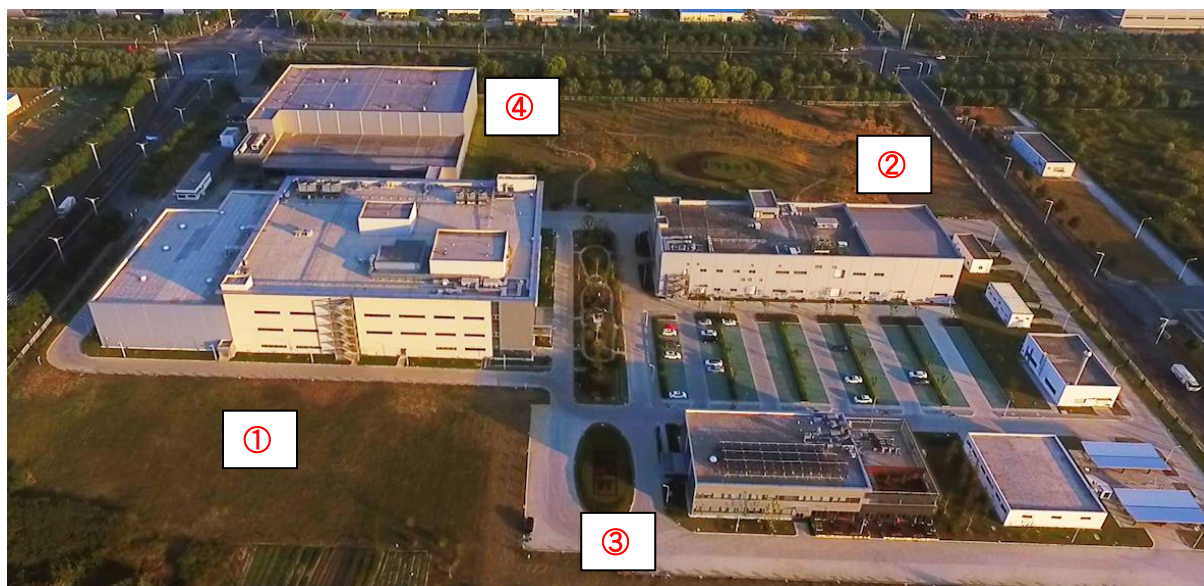
(Bird's eye view of the new Suzhou plant)
