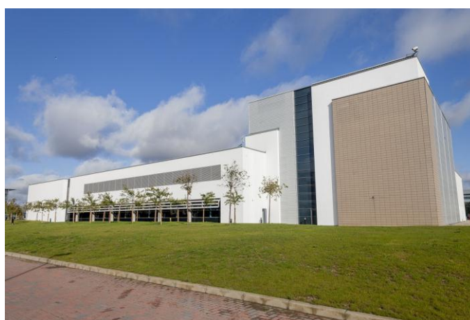
New Packaging Facility
